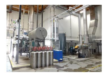
Utility systems instalation including new boiler, air compressors, and hot water generator.
