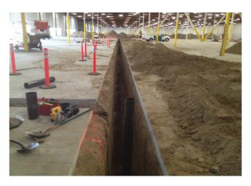
Installed 5,000 feet of Lab Waste CPVC industrial waste system piping fed by over 50 Stainless drain fixtures.
